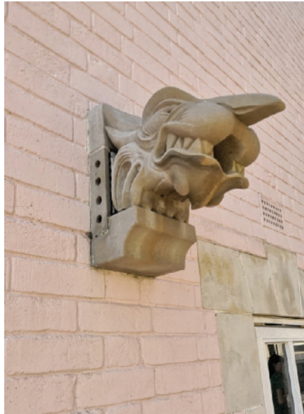
Figure 4: Gargoyle disguising boiler flue.
